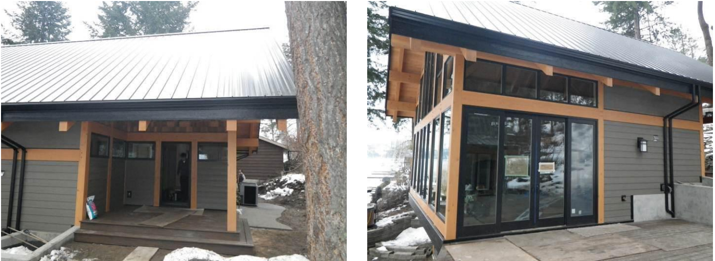
Fig.3.16 Air-tightness test house #3, Chase, BC.
