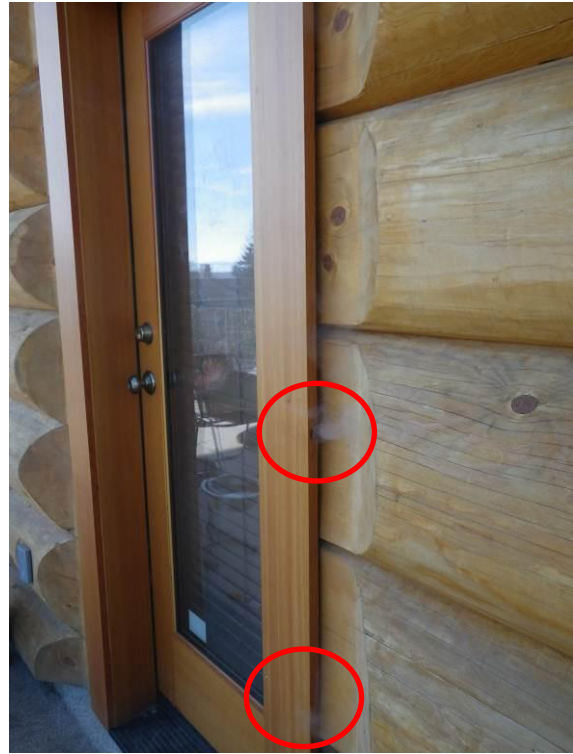
Fig.3.29 Smoke leakage observed at log wall corner joint (left) and at door (right) during pressurization.
