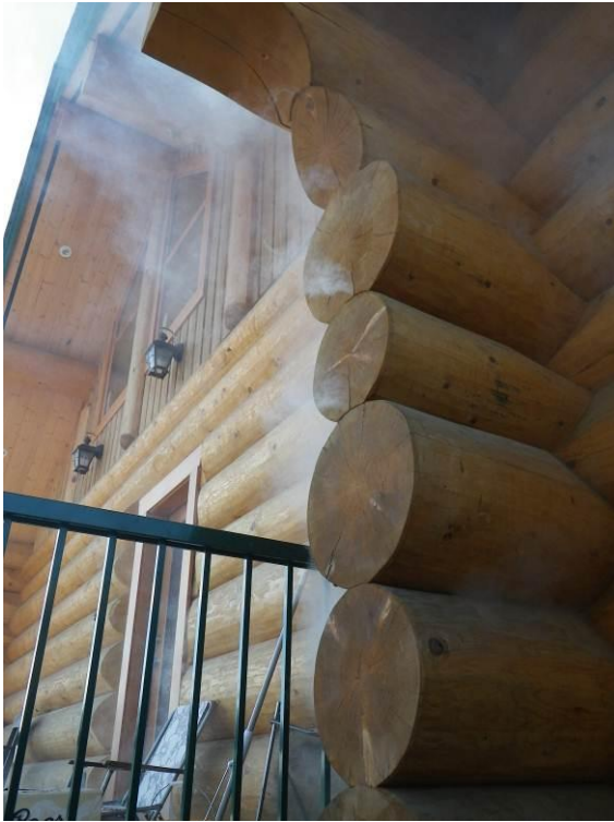
Fig.3.29 Smoke leakage observed at log wall corner joint (left) and at door (right) during pressurization.
