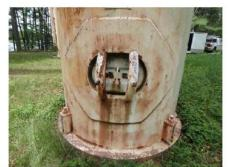
Shows riser manhole in very poor condition with heavy rusting.
