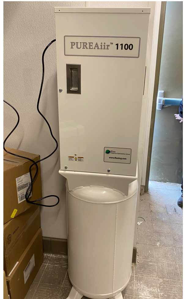
The PureAair and the storage tank can be remotely installed in separate locations.
