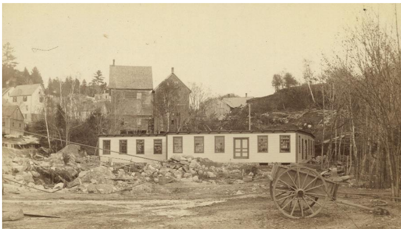
Pulp mill under construction, 1888. Site of Sunapee Village Dumping Station, 1903-1916.
