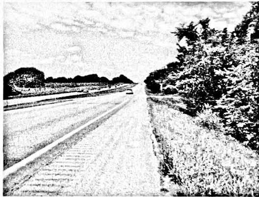
Facing west along subject's US-50 frontage
