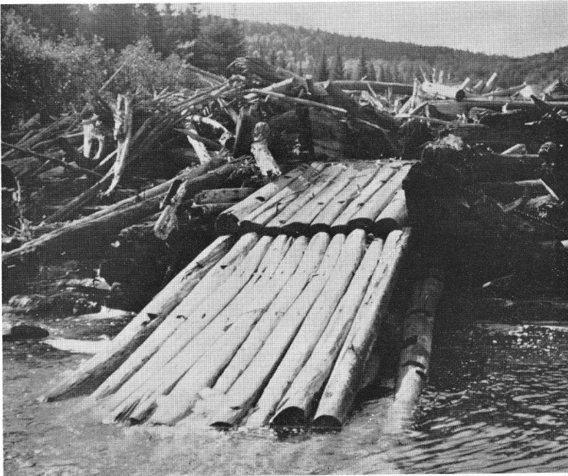
Figure 9. An abandoned log driving dam creating an obstruction to fish movement on the South Branch Birch River, T16 R8.
