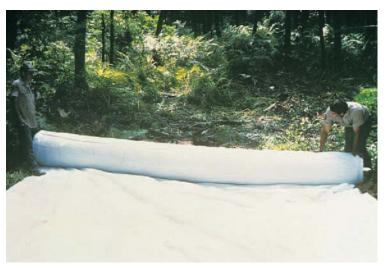
Use geotextile to keep fill from mixing with the wetland soil.
