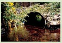
Culvert installed below the streambed level to allow fish passage.
