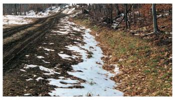
Revegetated road ditches carry water without eroding.
