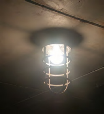
Photo 8: This light cover is insufficient to protect produce below from contamination in the event the light bulb breaks.
