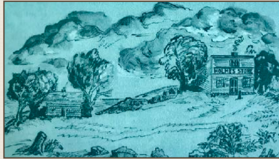
Holmes' original trading post and later store building, a pen and ink drawing by Lorraine Coller. From The Shakopee Story by Julius A. Coller, II, p. 27.
