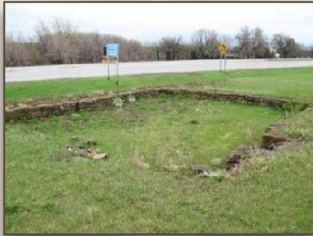
The wood frame Pond Mission House was razed in 1907. The foundation is still there, across the road from Memorial Park in east Shakopee. A historic marker tells about the Mission House and Reverend Samuel W. Pond.
