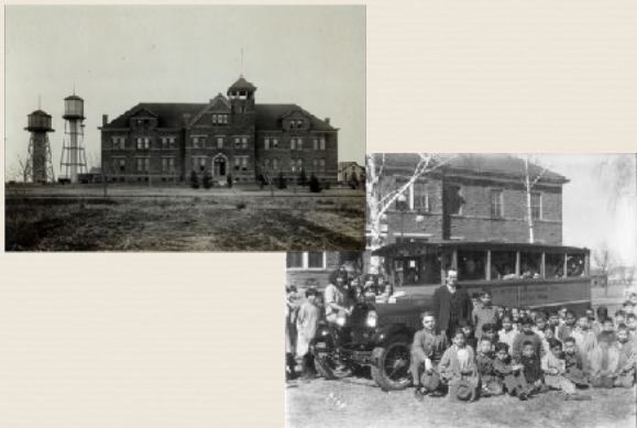
Pipestone Indian School in Pipestone, Minnesota, where Rosemma Coursolle attended school. Chester E. Sogn, Pipestone Indian Training School students, Pipestone, Minnesota. 1893 - 1953. Pipestone County Historical Society, collection.mndigital.org/catalog/pipe:158 Accessed 22 Feb. 2022.
