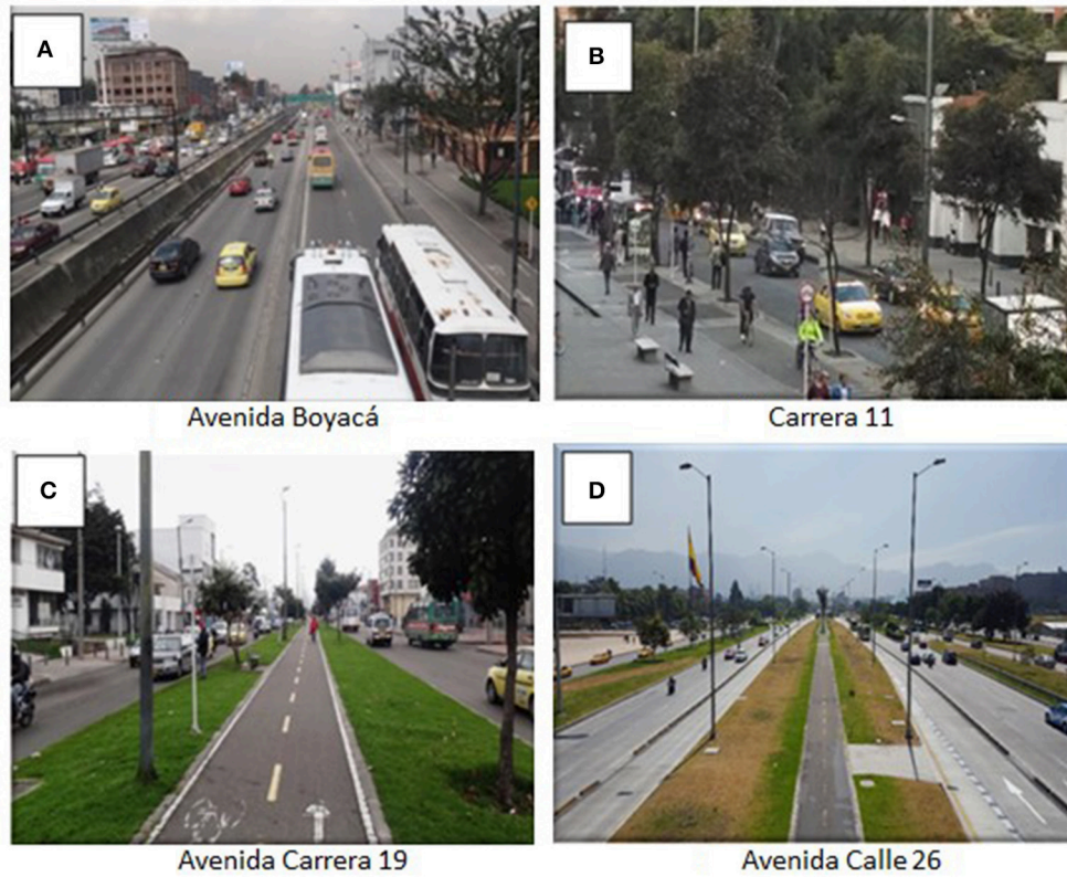
FIGURE 1 | Configuration of the streets and bike-paths selected for this study. (A) Open street with lateral bike-path; (B) closed street with lateral bike-path; (C) closed street with central bike-path; (D) open street with central bike-path.
