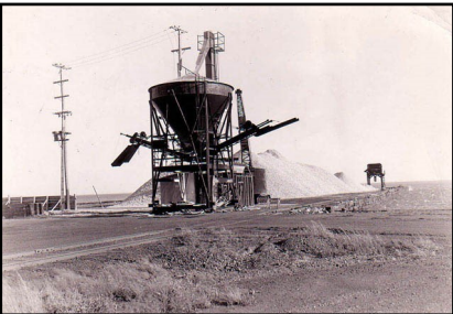
Grain hopper at commercial dock
