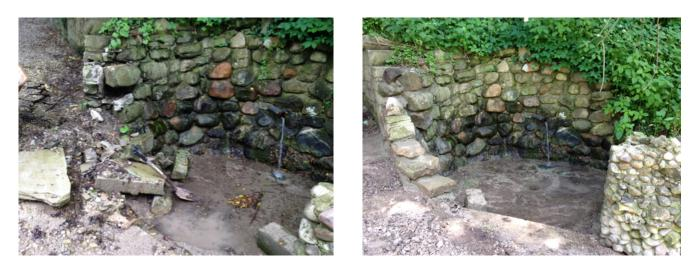
properly operating, weekly, and regular trash pickup, has been integral for the positive outward appearance of the historic site, around which Amherst was founded. Another task has included re-mortaring stones and restoring concrete steps (before and after views above). Ultimately, this area must continue to be honored and maintained as such.
