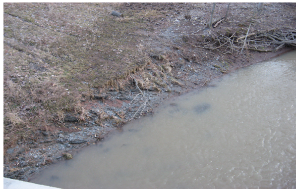
Stream bank erosion as a result of nonexistent well-vegetated riparian buffers along the Beaver Creek stream bank.
