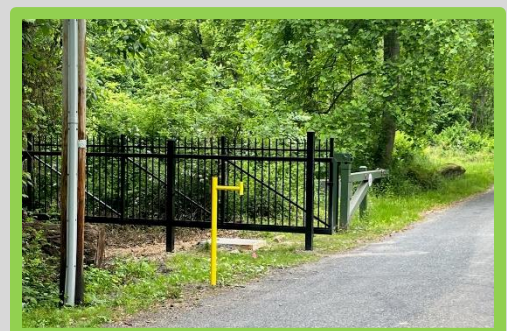
Photo courtesy of Bob Walker
