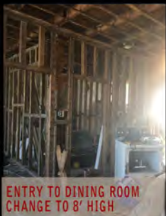
FRAME HAS BEEN INSTALLED FOR POWDER ROOM AND LAUNDRY ROOM
