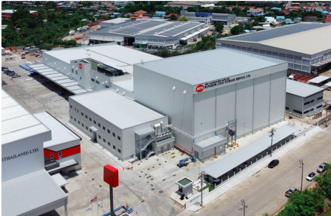
[Exterior View of the New Warehouse]
