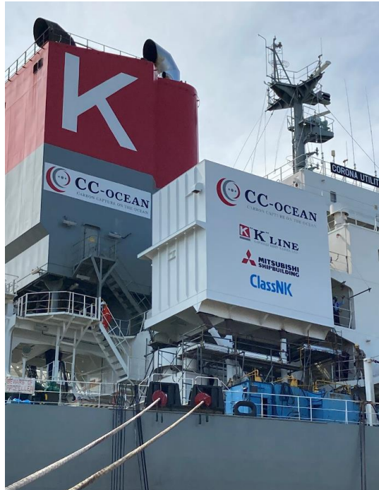
4. Installing on vessel ②
