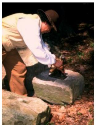
Living history programs are staffed by Park Service employees and volunteers on some weekends. Here a stone mason shows how holes for mounting cast iron chairs were marked and hand-drilled in a stone sleeper. The thousands of stone sleepers used in construction of the levels on the Allegheny Portage Railroad, including this one, were quarried directly from limestone out croppings that lined the route.
