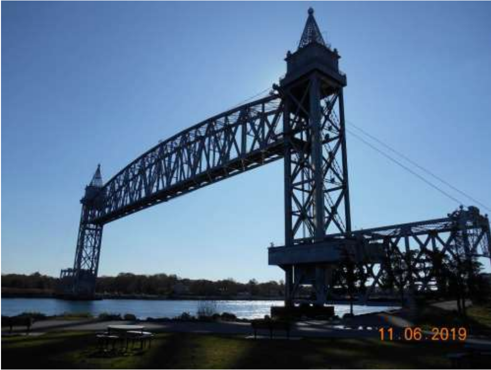
Fig. 17 Cape Cod Canal Vertical Lift Railroad Bridge
