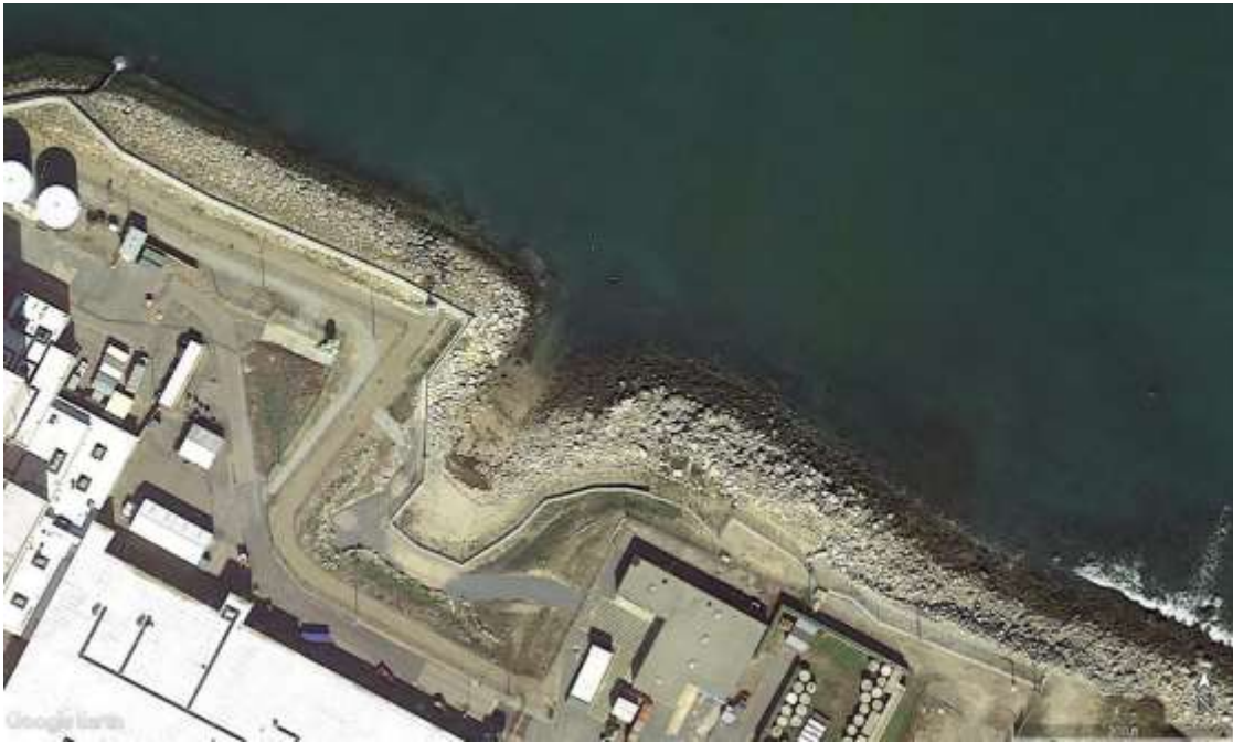
Fig. 12 Aerial view of barge access at the Pilgrim site
