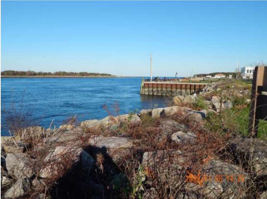
Fig. 15 First potential barge to heavy haul truck to rail transload location
