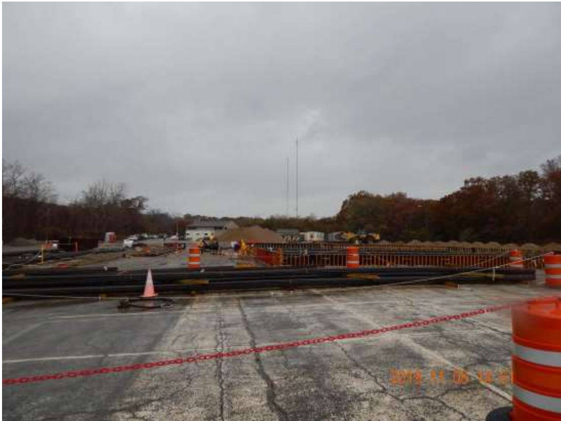
Fig. 4 Construction of new Pilgrim ISFSI
