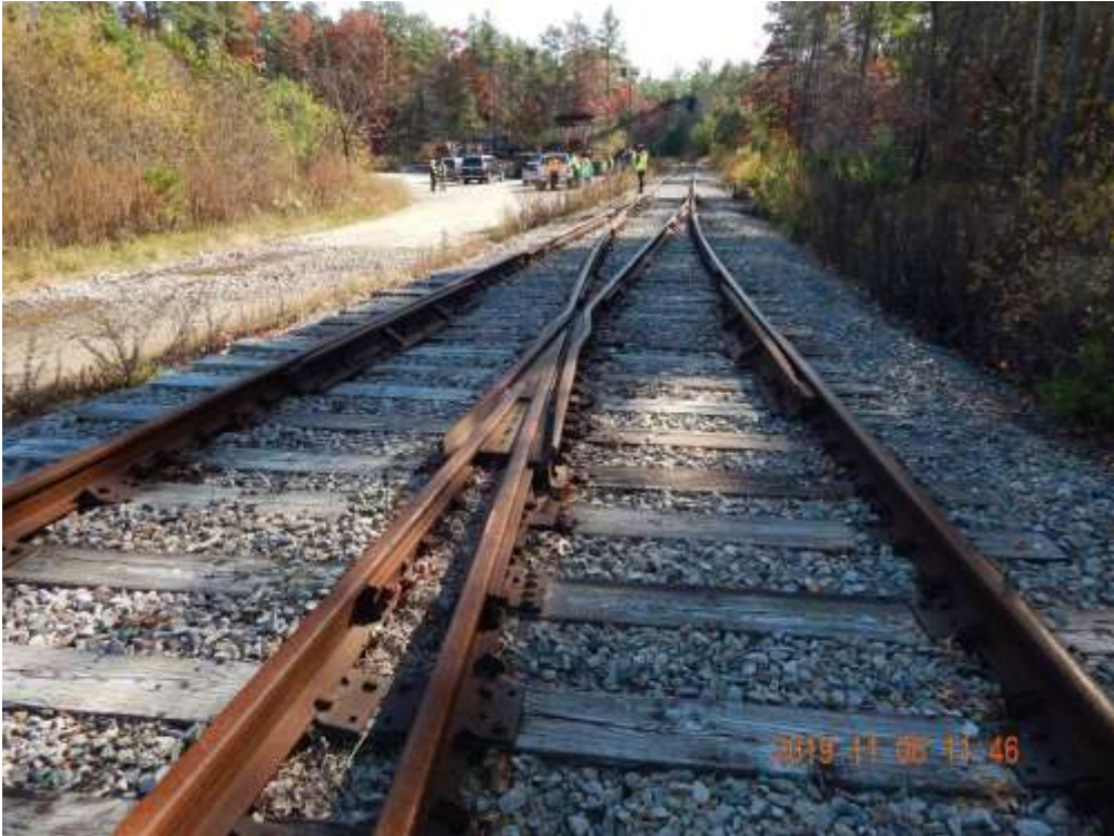
Fig. 9 Second potential Middleborough, Massachusetts transload location (looking south)
