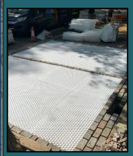
Not only are these new spaces a little wider to help reduce door bumping but also the mesh-gravel combo is completely porous allowing for much better water drainage. The recent flood saw large amounts of water draining away through the gravel as it over ran the car park's gutters.
