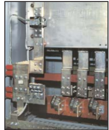
Fig. 16: Rear views showing ground fault protection with ground and neutral disconnect links
