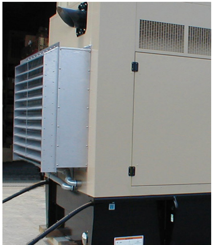
Figure 3: A 200 kW resistive load bank mounted on the radiator of a generator set.
