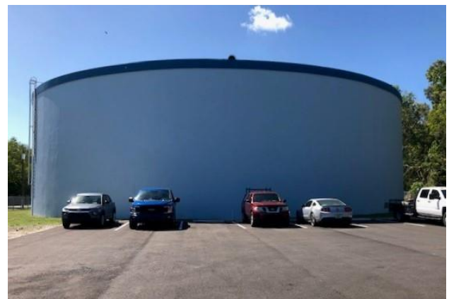
Repainted 3-million-gallon storage tank at Center.
