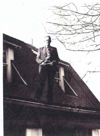
Bill W. on the roof at Stepping Stones
