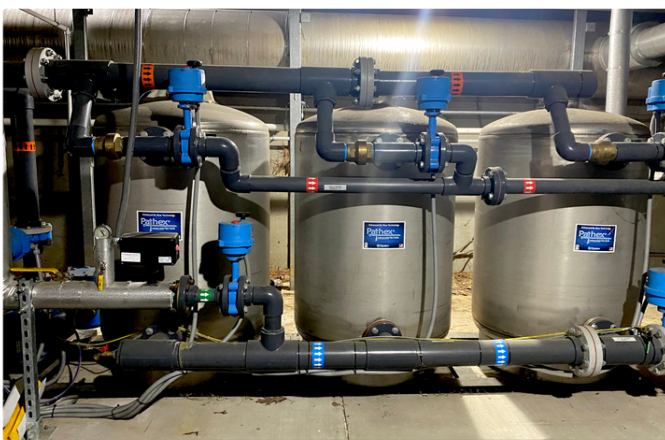
Triple 36" side stream filter system containing PathEx antimicrobial filter media
