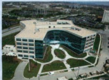
Finalists for SSI's 2009 Integrated Installation of the Year included (top to bottom) Advanced Technologies, CRS Building Automation and Stanley CSS.
