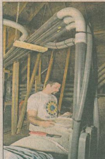
Thomas Marino looks over schematics and design printouts of an automated system he is installing in a house off Highland Road. The conduits surrounding him will lead wiring from all over the house to a main control panel.
