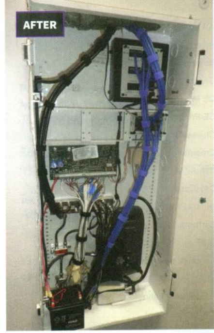
Advanced Technologies' cleanup for this security-centric job included tidying up the wires and cables and moving the modem and router from the enclosure to the shelf above. Company president Tom Marino says that enabled them to install and close the panel cover, which was not done (and not possible) before.
