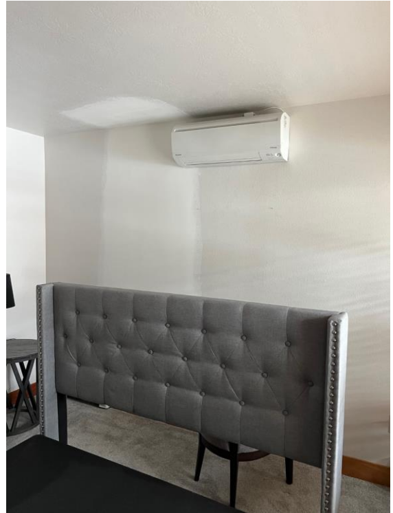
Downstairs with Wall Patch (Pre-texture and paint)
