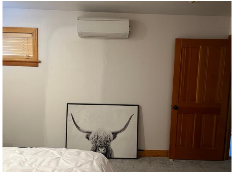
Upstairs with Wall Patch (Pre-texture and paint)
