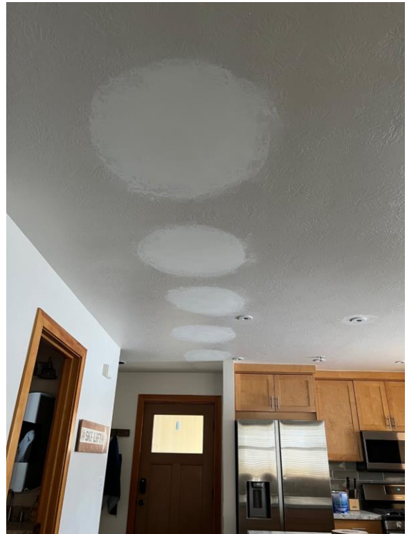
Kitchen Ceiling Patch (Pre- texture and paint)
