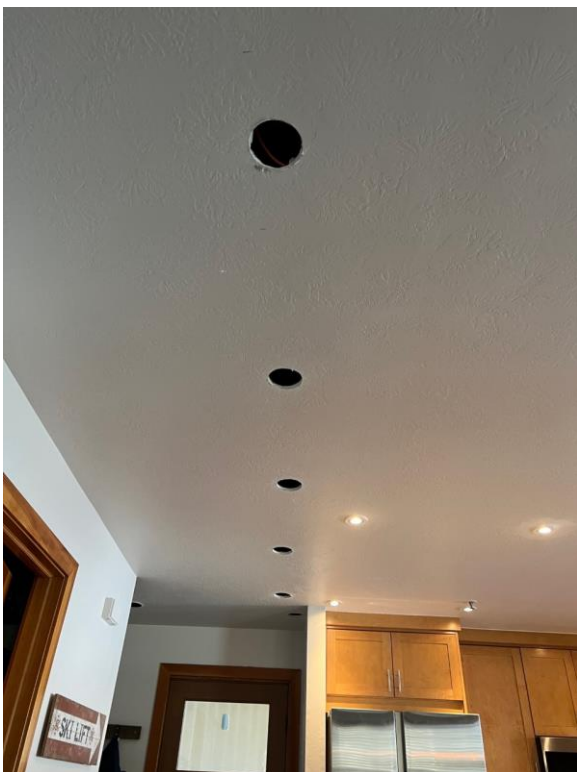
Kitchen Ceiling Fishing Holes for AC Power
