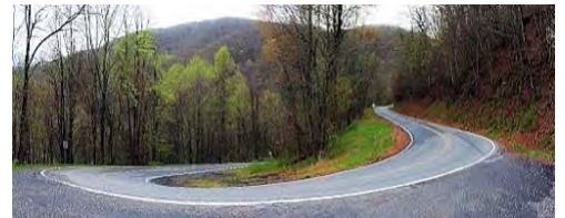
Many switchbacks along Wayah Road
