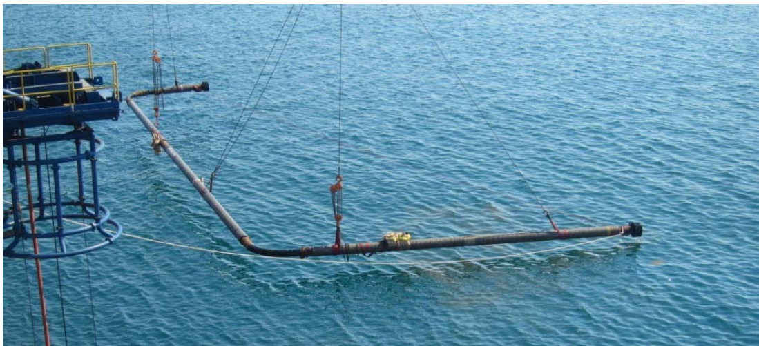
Figure 5-3 Example Expansion Loop Spool (Saka Petroleum)
