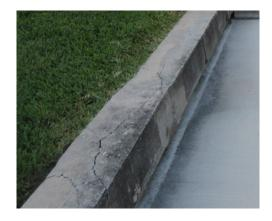
As you can see, there is cracking, spauling, and exposed rebar, and it is this type of damage that can be inexpensively repaired, compaired to complete replacement.
