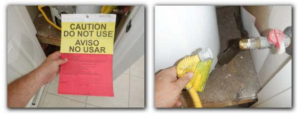
Located in house without benefit of a drain pan. Should water heater leak interior flooring can be damaged REF.: 1991 Standard Plumbing Code 1213.7.1 IRC 2801.5.
