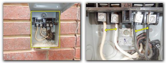
The southern A/C disconnect box was observed to be rusted / damaged.
