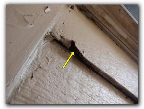
Evidence of possible wood destroying insect damage observed in the garage; Final determination of structurally significant damage to wood members cannot be determined without removal of wall covering {interior sheetrock or exterior siding}.
