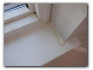
Possible from exterior window frames not properly caulked / sealed.
