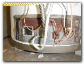
Corrosion observed at shut off valve and/or connections on top of water heater.
