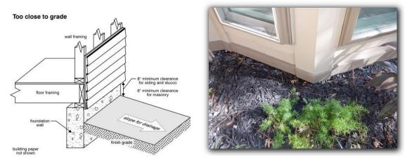
Soil level too high, or close to Hardi plank siding, promotes wood rot and is considered a conducive condition to termite activity at one or more locations around house/garage.
