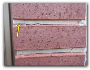
Caulking deficient around one or more windows, will allow water penetration during heavy / wind driven rains.
