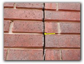
Uneven separation of expansion joint was noted between the upper and lower wall at the east exterior.
