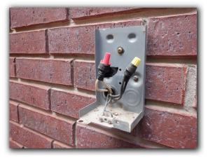
Protective bushing not present around electrical wire as it passes through metal box of the northern A/C disconnect.
