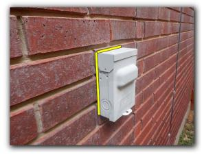
Expansion joint(s) and / or inside corners in brick veneer need caulking. Ensure any mortar present in expansion joint is first removed before sealing.
