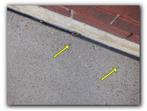
Caulking missing and/or deficient around vertical trim boards may allow wind driven rain entry.
