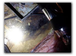
Secondary drain pan is rusted; indication coil (or previous coil) has history of leaking/dripping condensation into pan.
