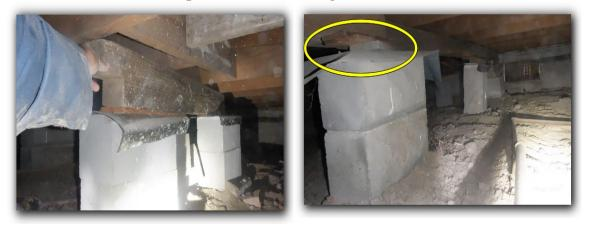
Wood deterioration to a foundation perimeter beam can be observed at the back yard, recommend having the beam replaced if possible for structural integrity.
