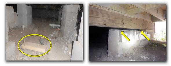
Crawl space ventilation is limited. Conducive condition for wood rot and mold if not corrected. Only 1 foundation vent observed on the front part of the house and none on the east side of the structure. Cross ventilation throughout the structure should be present.
