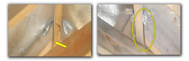
Some disconnection of the purlin and rafter observed on the north side of the older attic section. This is the older attic and appears to have some expected sagging or out of square framing. The new purlins due to this condition were some what disconnected.
