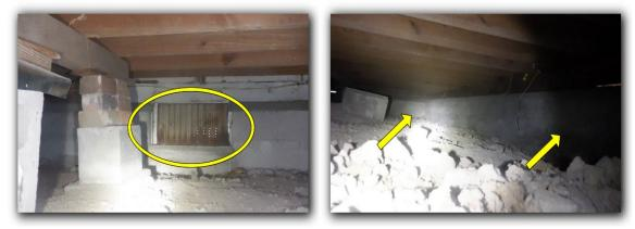
Observed wood framing under house has inadequate clearance from soil to prevent wood rot according to code. Minimum soil clearance to untreated wood joists is 18". Minimum soil clearance to untreated wood beams is 12". IRC R317.1 (multiple locations)
