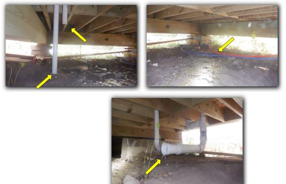
Note: old cast iron drains and galvanized plumbing observed, recommend removal of all unused antiquated plumbing to prevent giving the perception that the plumbing is still active should be future inspection occur.
