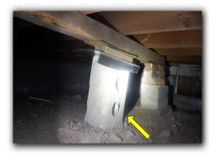
Scrap wood below house is considered a conducive condition for wood destroying insects. A beam at the east/central location is not properly supported or chimmed.
