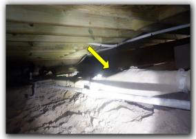
Note: old electrical wiring observed, recommend removal of all unused antiquated wiring to prevent giving the perception that the wiring is still active should be future inspection occur.
