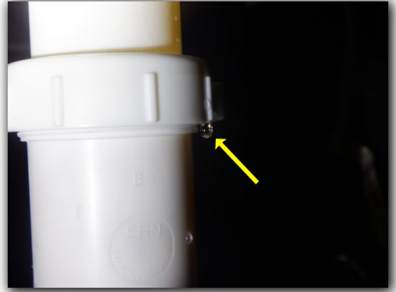
Small leak below sink, (Northern 2nd floor bathroom sink)
