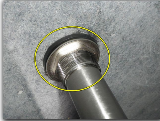
Small leak below sink, (Northern 2nd floor bathroom sink)
