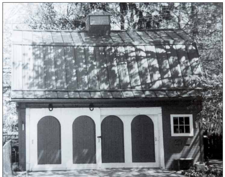
Barn with metal clad roof and original hardware.
