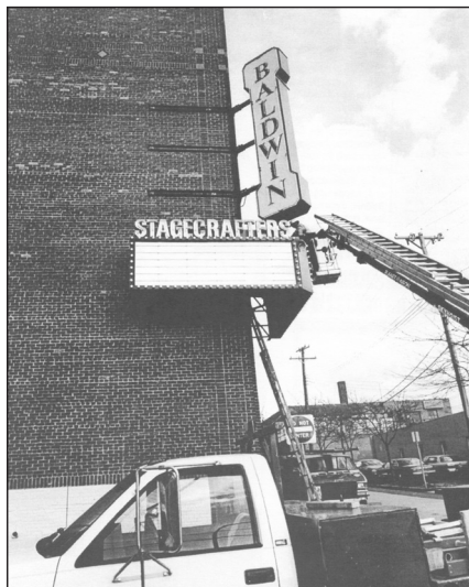
The current marquee being installed in 1996.
