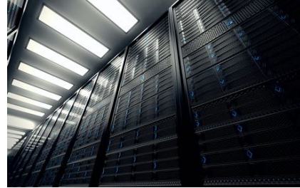
Servers (Cloud computing)
