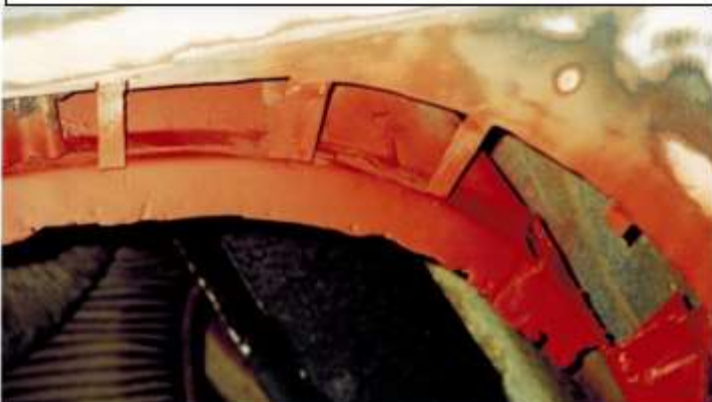
Fabricating metal tangs offset to receive & support fiberglass patch panel in 2001
