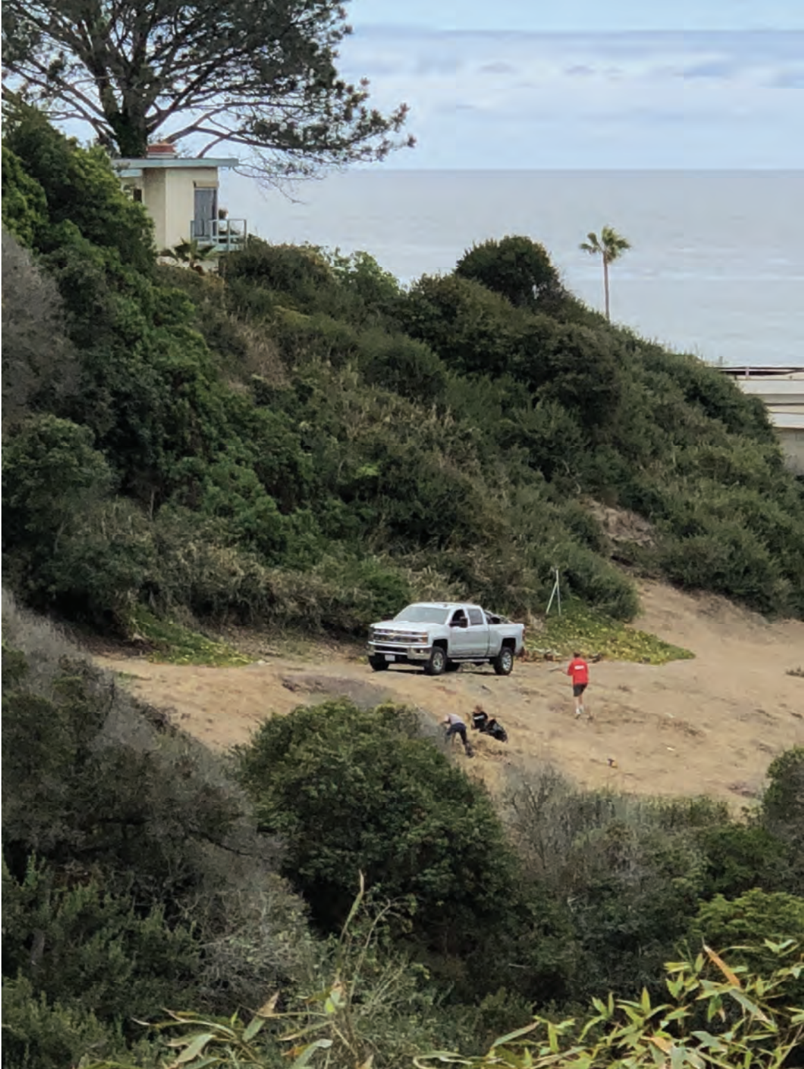
Figure 1c. Photo showing clearance of the site.
