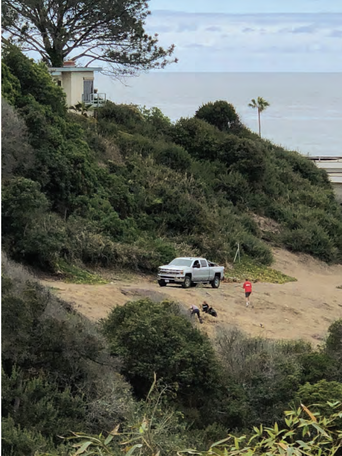
Figure 1c. Photo showing clearance of the site.
