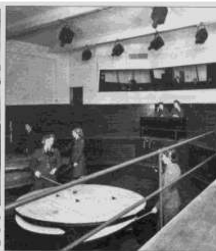
Reporting Room of final GCI station, AMES Type 7, generally known as the Hap.
