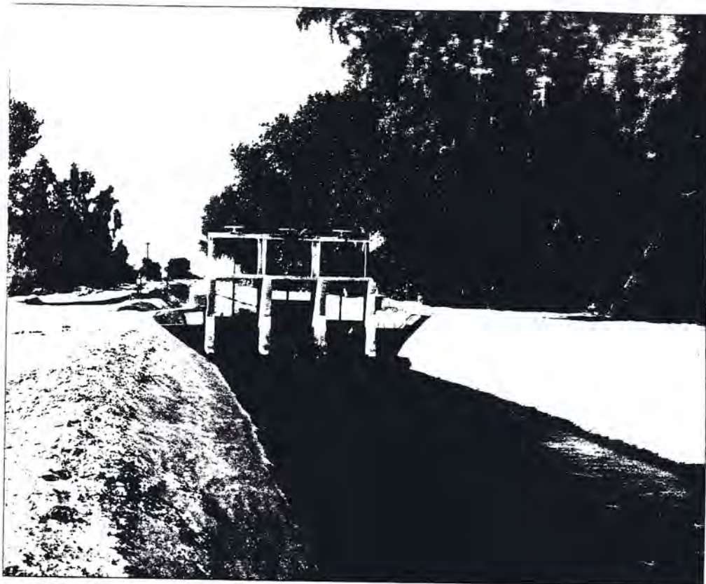
U.S. and Mexican irrigation canals show that water delivery systems will influence competing agriculture in the two countries. Above, a concrete canal in Imperial County reduces water loss due to soil percolation and weed competition, in contrast to the Mexicali gate ditch canal below. Soil salt buildup is also a more severe problem in Mexico, where there is no equivalent of Imperial Valley's subterranean tile drain system.
