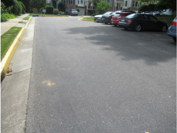
Asphalt pavement overview
