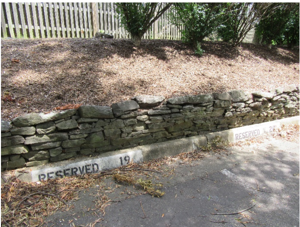
Landscape stone retaining wall overview
