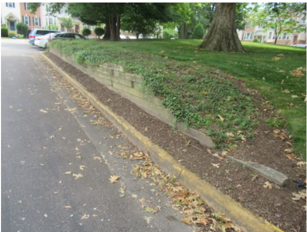
Timber retaining wall at Peter Roy Court overview
