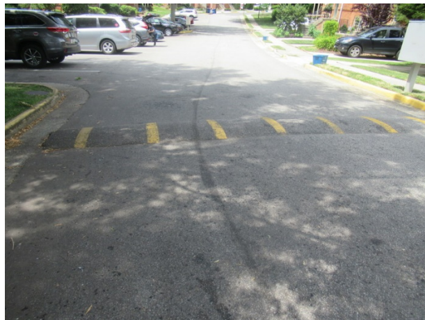
Asphalt pavement and speed bump overview
