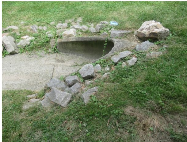
Concrete inlet structure overview
