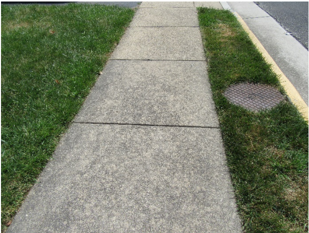
Concrete sidewalk overview
