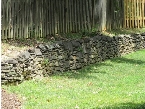
Landscape stone retaining wall overview
