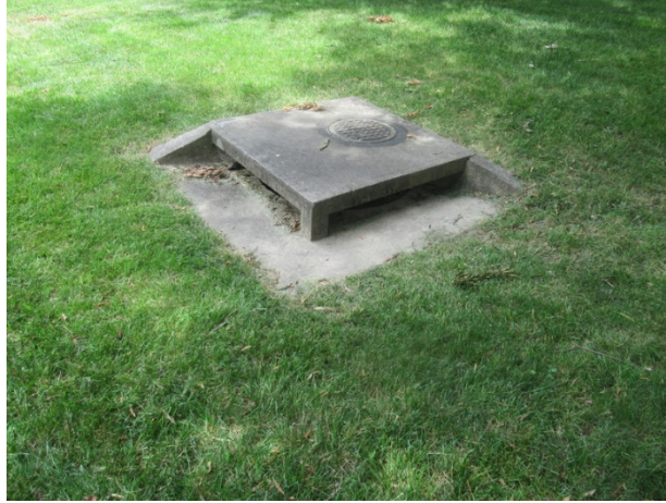
Landscape catch basin overview
