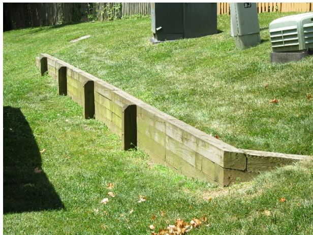
Timber retaining wall near 9433 William Kirk Lane overview
