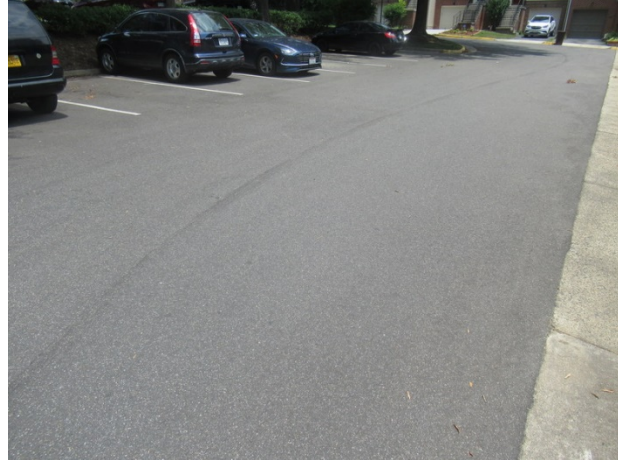
Asphalt pavement overview
