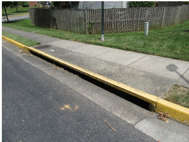
Catch basin overview
