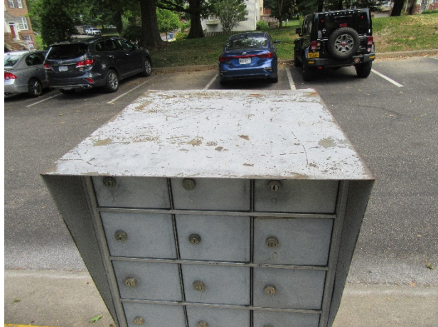
Finish deterioration and rust – Note: original station
