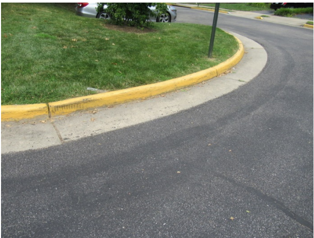
Concrete curb and gutter overview
