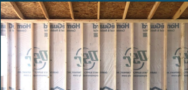
HOUSE WRAP VAPOR BARRIER | P1
