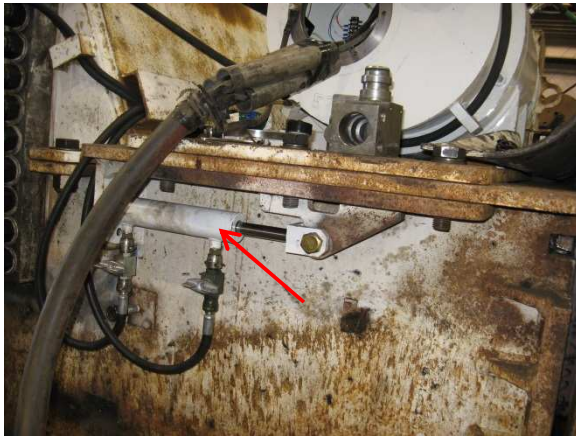
Figure 44. Crusher Motor Belt Tension Adjustment Using Hydraulic Cylinder.
