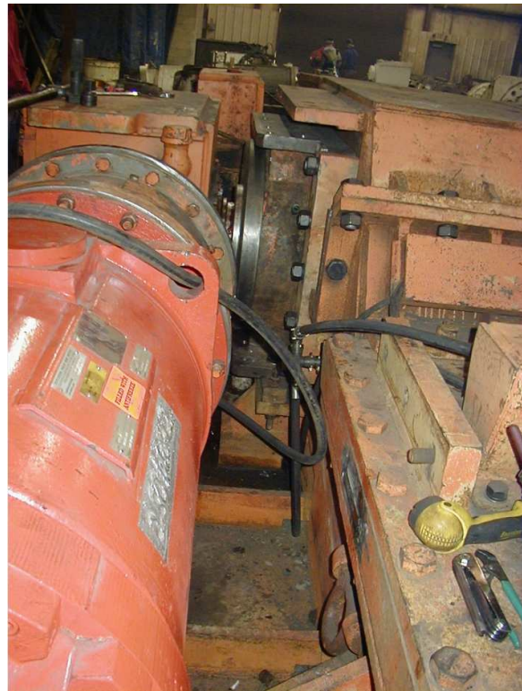
Figure 49. View Along the Motor Looking At Gearbox/Crusher Shaft Mounting.
