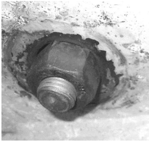
Figure 35. Motor Hold Down Bolt, Corners of Nut
