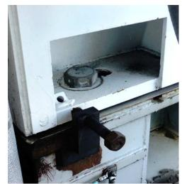
Figure 8. ID Fan A & B Motor Hold Down Bolts Used Tapped Holes in Fabricated Steel Base.
