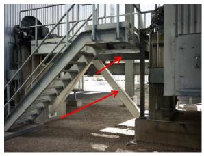
Figure 3. ID Fan A & B, Outboard Pedestals, Steel Bracing Bolted to Each Pedestal.
