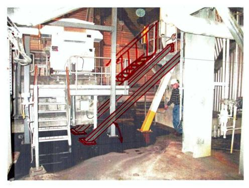
Figure 37. FD Fan A OB Pedestal Bracing and Platform Access by Stairs Modification.
