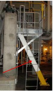
Figure 4: ID Fan A Outboard Bearing Pedestal Single Brace 30 Deg Angle.
