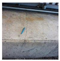
Figure 5. ID Fan A Foundation Crack.
