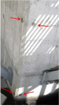
Figure 18. ID Fan A Outboard Pedestal With 410 SS Targets Epoxied.
