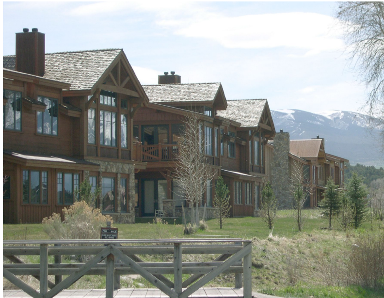
Buildings #1 & #2 Photo from 2005
