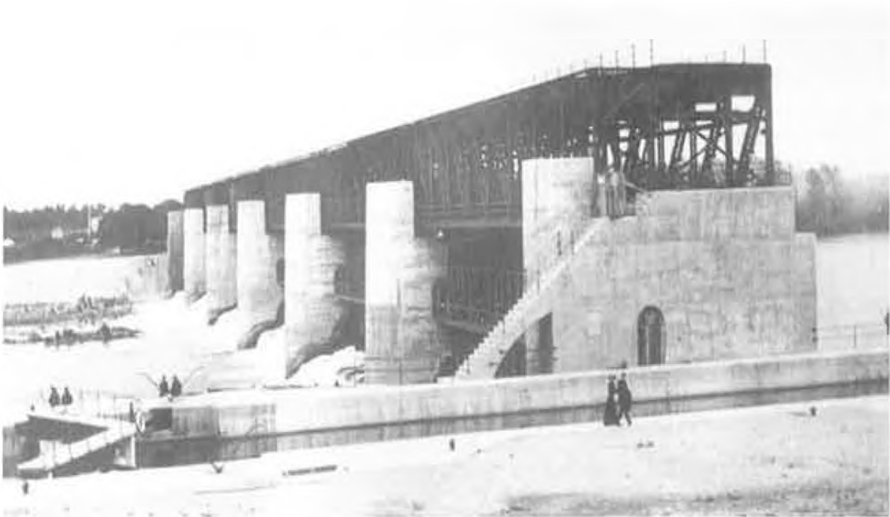
The lock and dam soon after its completion in 1910. The roadway decking and approaches have yet to be constructed at the time of these pictures. Note the people fishing on the downstream side. (Manitoba Archives Photo.)
