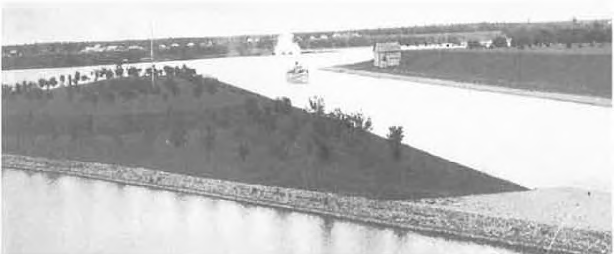
Views of the upstream approach to the lock, taken from the bridge and from on board an excursion steamer. The concrete abutment at centre acted as an ice breaker during the spring melt to help minimize damage to the structure as the ice flows passed through the open dam gates. Although the old time steamers are long gone, boating excursions are still popular. The Island was created from mud from the base of the dam.
