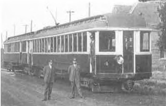
In front of the Selkirk Ticket office next to the current Selkirk Lift Bridge
