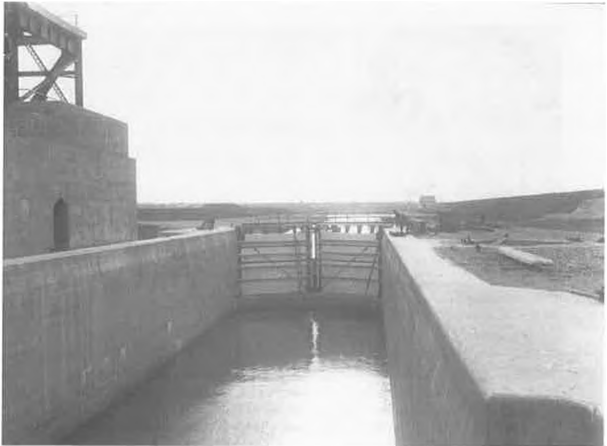
The Lock portion was constructed June-October 1907 The total construction materials for the total project –The Lock is 215 ft and 45 ft wide with a 17 ft lift at normal water levels and a maximum lift of 22ft at low water levels. It can accommodate vessels of 1600 tons (Lord Selkirk)
