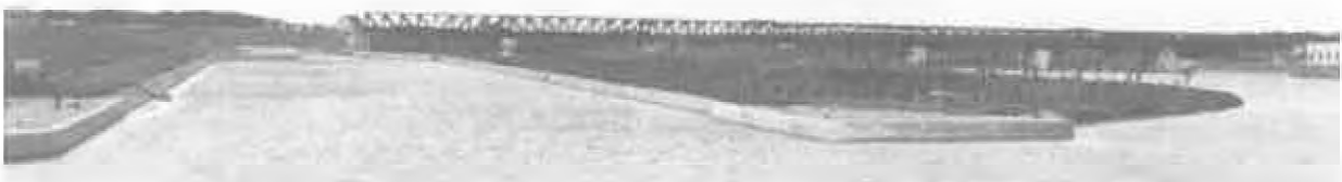
Views of the upstream approach to the lock, taken from the bridge and from on board an excursion steamer. The concrete abutment at centre acted as an ice breaker during the spring melt to help minimize damage to the structure as the ice flows passed through the open dam gates. Although the old time steamers are long gone, boating excursions are still popular. The Island was created from mud from the base of the dam.
