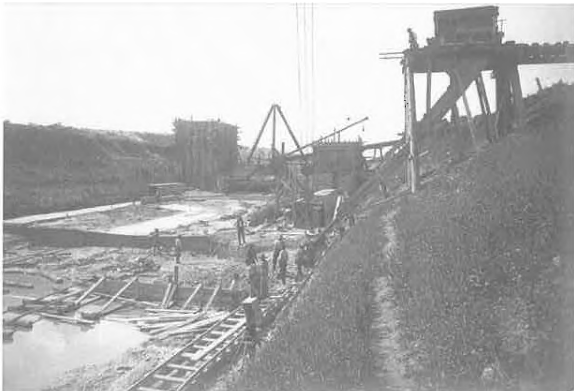
A view of construction work being undertaken at lock site. Much of the excavation work was undertaken by manual labour and teams of horses dragging “Fresno” scoops. (Manitoba Archives Photo.)
