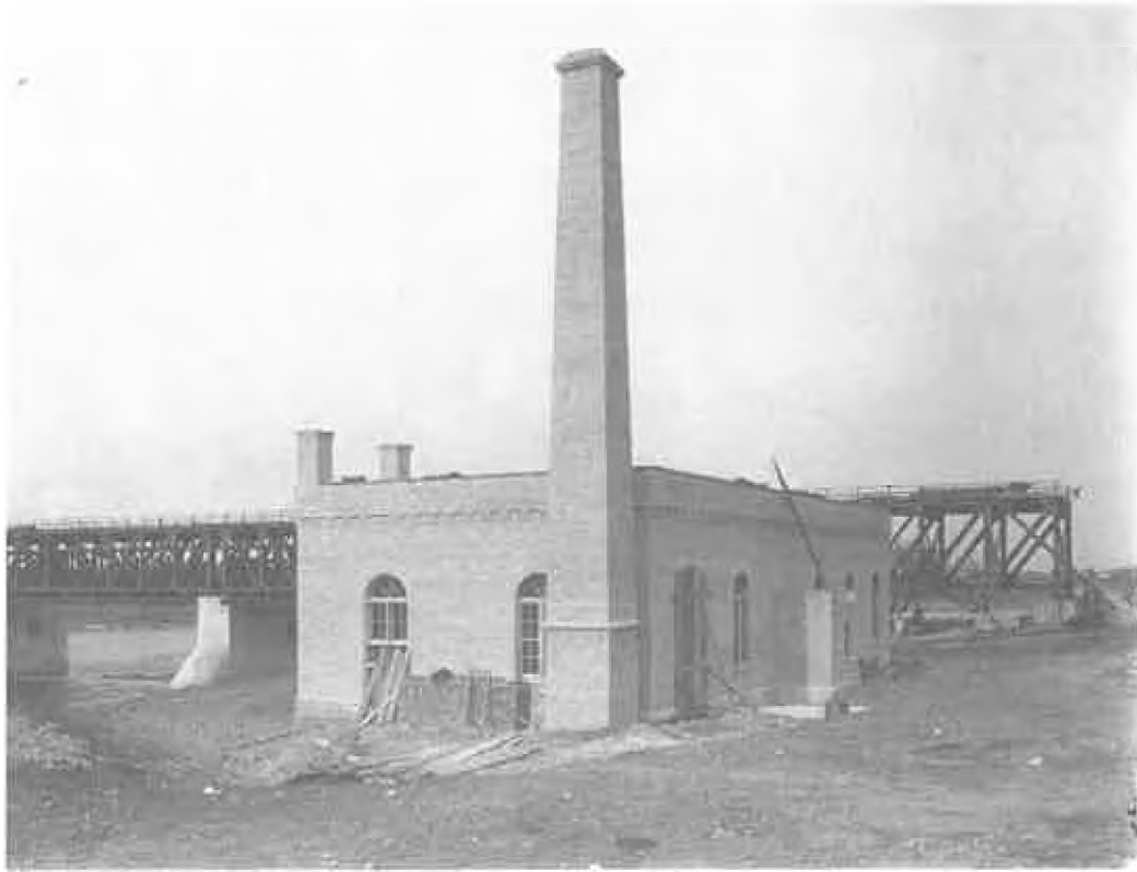
The repair shop and power house for auxiliary electric power, however power was never needed as electricity was purchased from Winnipeg Electric Co. in 1923.
