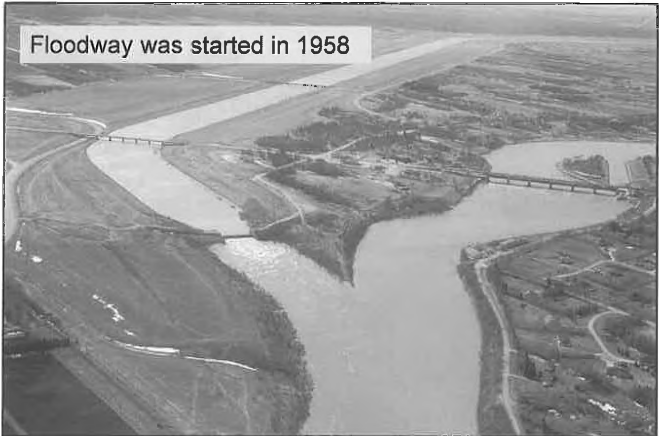
Red River Floodway outlet located just downstream from the Lockport Bridge and Dam. In this photo, the floodway has been opened during the spring melt. Normally the floodway channel would contain a trickle of water, particularly during the summer and autumn when river water levels are naturally low.
