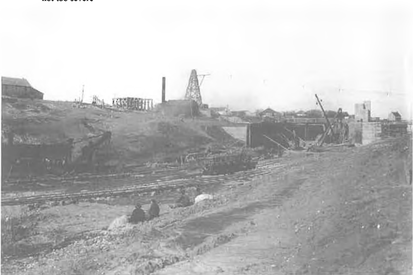
Spur rail line from the Selkirk Branch for the purpose of moving heavy machinery and materials
