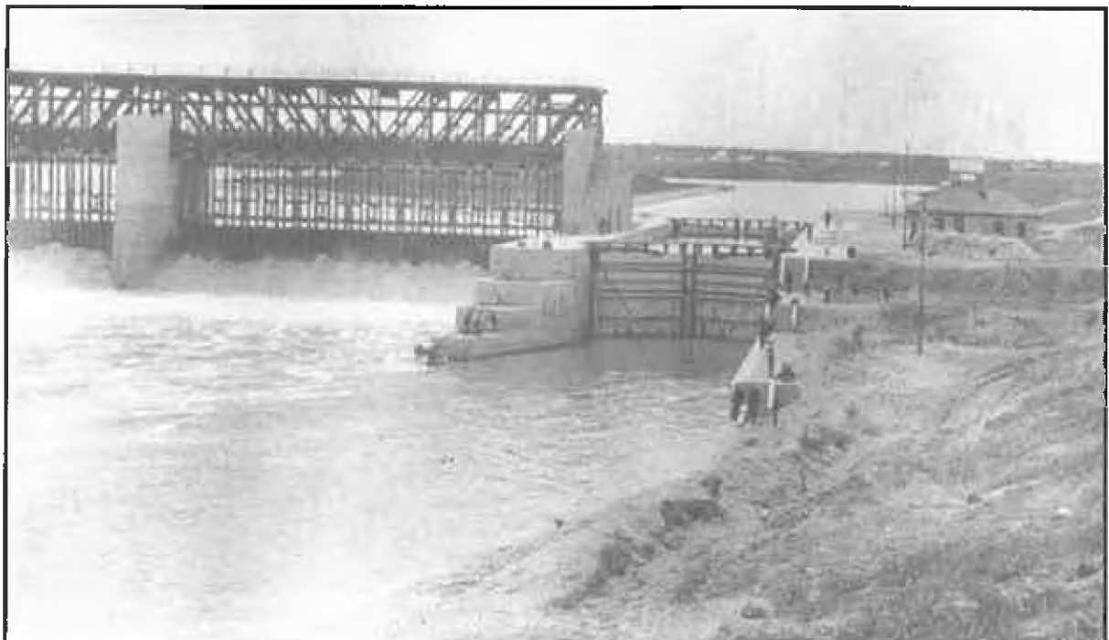
Lock design was very modern for its time with automatic self-balancing valves so the lock could be filled and emptied by a 4.5ft x 6ft culvert sluice located at the base of each side wall and opening into the lock chamber through a series of 8 ports At the time the four sluice “Cluett” automatic lock valves were the largest in the world
